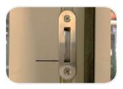
SECURE THE HOOK KEEPER TO THE JAMB.
