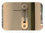
LINE UP THE BOTTOM KEEPER ALLOWING 1/8 INCH GAP FROM YOUR LINE TO THE TOP & MARK THE HOLES.
