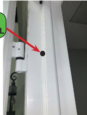
7. Cross tape your frame to make sure your frame is square and use a level on the jamb to make sure it's plumb. **(Fig. C)**
